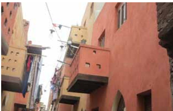
A house after restoration © Mona Zakaria Architects
