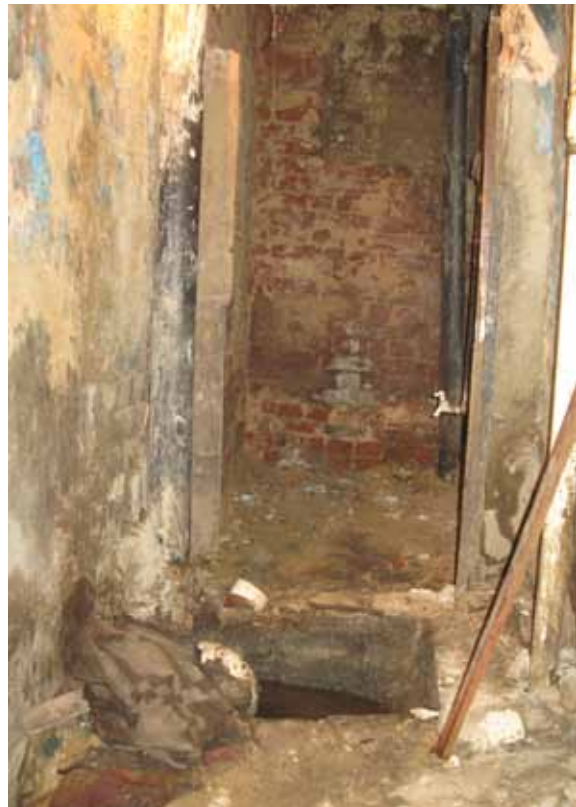
'Toilets' before improvement work © Mona Zakaria Architects
