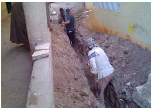
Excavation work © Together Association
