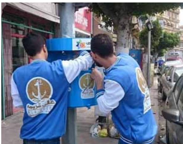
New waste bins being installed © Port Said 'Ala Qadimoh
